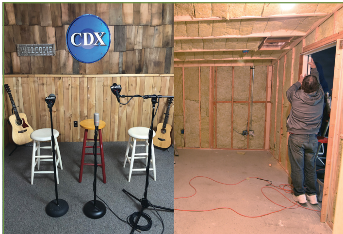
2020 bringing new looks! We've renovated our video studio (left) and the CDX recording studio (right) is under construction!
